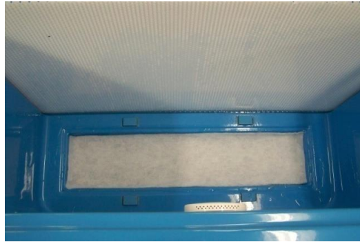
Figure 3: showing a media pad laying on top of the bottom grate.
